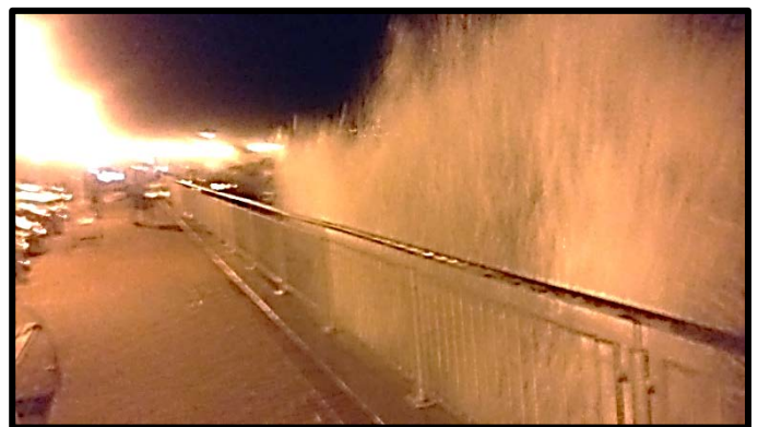
"Waves' spray at St Clair Seawall"
